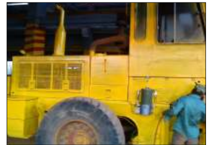
#2050 POLYHYB - BEING SPRAYED - ON USING HVLP GUN
